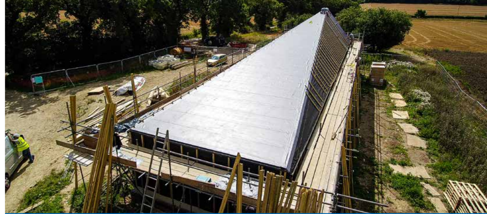
DANOPOL® WATERPROOFING COMPLETED
